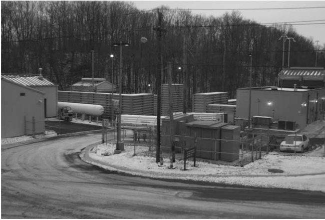
Fig. 1. The Creek Road Complex. The SMiRF test building is shown on the right. The shop building is shown on the left. The roof of CCL-7 is visible behind the barrier walls at the left.
