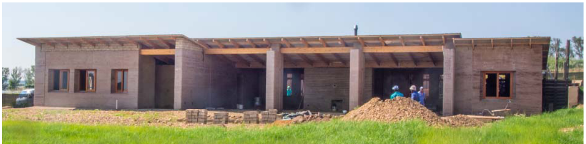
Figure 1 North View of rammed earth house
