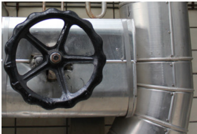
Fig. 1 Example of insulated oil pipe using mineral wool and sheet metal cladding.
