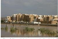
Figure 2: Yemen high rise towers made of mud bricks [7]
