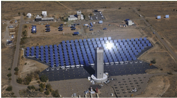
Fig. 1. Sandia's concentrating solar power tower at the National Solar Thermal Test Facility, Sandia National Laboratories, Albuquerque, NM.
