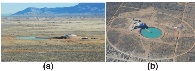
Fig. 1. Large-scale LNG facility: (a) side view and (b) top view.
