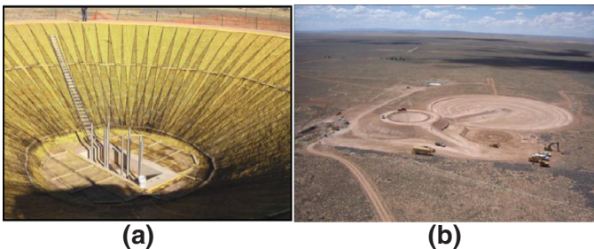
Fig. 2. Reservoir construction (a) and water pool excavation (b).
