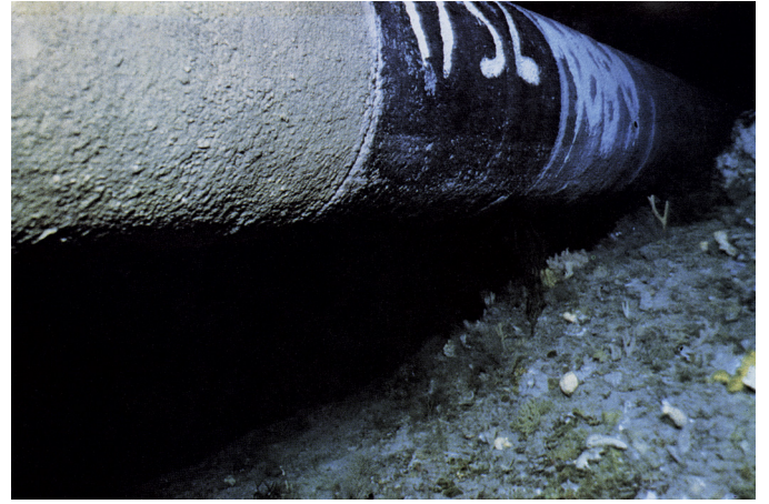
Fig. 1. A free spanning concrete coated pipeline (photo: DNV GL).
