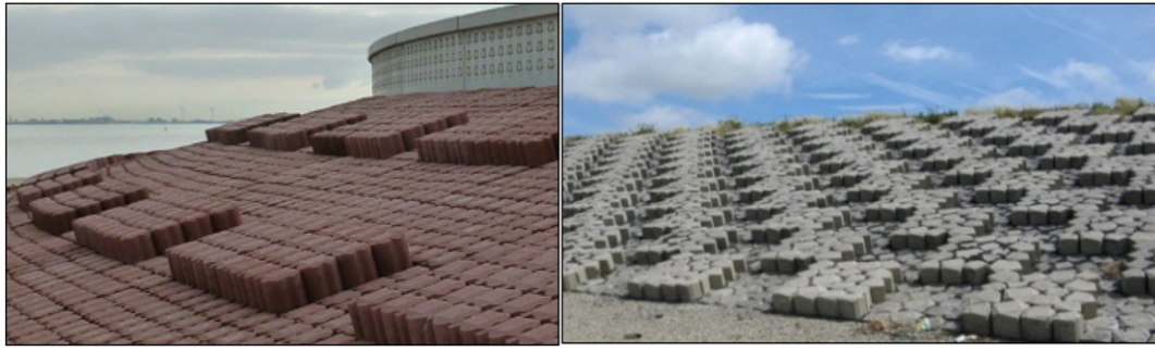
Fig. 1. Rib pattern Hydroblock® block revetment (left) and chessboard pattern Basalton® block revetment (right).
