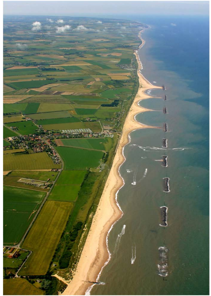
Fig. 1. Aerial photograph of the Sea Palling scheme, looking northwest, (courtesy of Mike Page).
