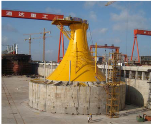
Fig. 1. Photograph of a composite bucket foundation.
