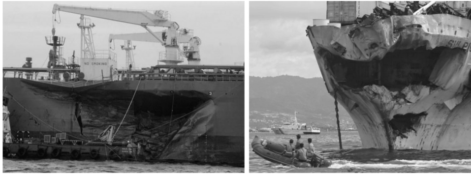
Fig. 1. Collapsed structures after ship to ship collision accidents occurred in the Singapore Strait (2010) and in waters of Talisay City, Phillipines (2013).
