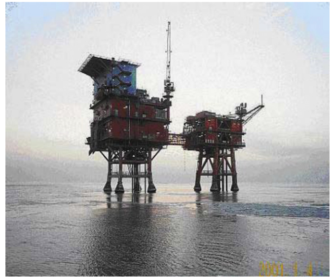
Fig. 2. Multi-leg jacket platform of JZ20-2 oil field.
