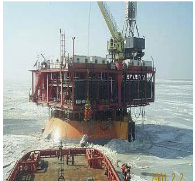
Fig. 3. Caisson platform in JZ9-3 oil field.
