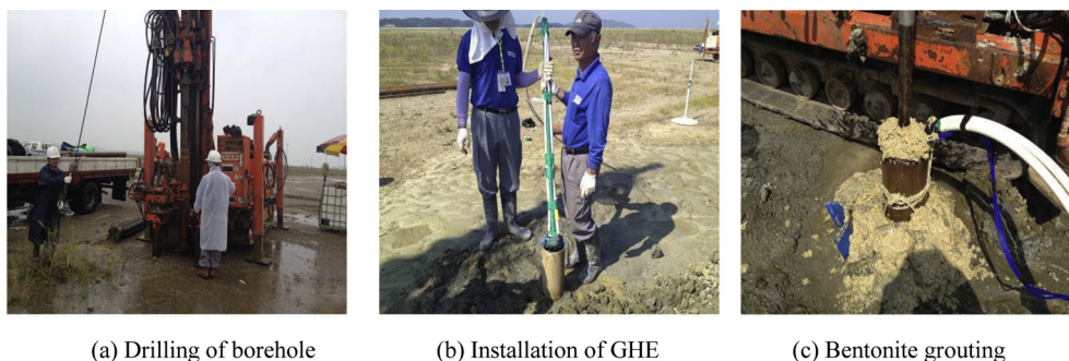
Fig. 2. Construction process of GHE.
