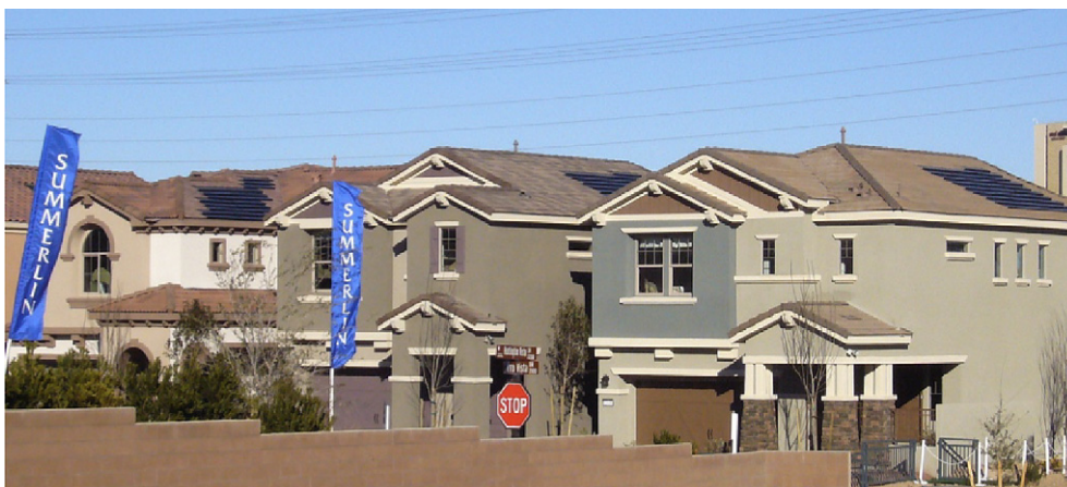
Fig. 1. Model homes built as a part of the proposed energy efficient residential community.
