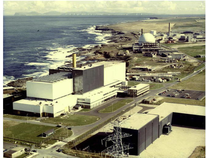
Fig. 1. PFR overall survey.
