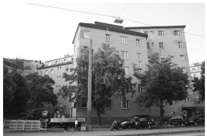
Fig. 1. Elderschhof Housing Block, Elderschplatz 1–2, 1020 Vienna, 1931, Architect: Ludwig Davidoff.
