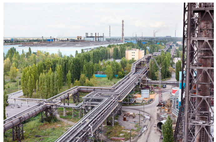
District heating: A pipe network that allows centralised heat sources to be connected to many heat consumers (Image courtesy of Shutterstock).
