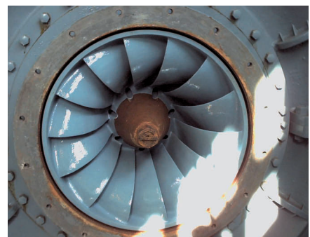
Figure 6. Completed runner installed and ready to return to service.
