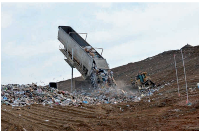
“An enormous amount of solid waste is dumped in landfills, such as the Palmetto Landfill in South Carolina which produces waste methane gas that can be utilized to create bioH 2 for use in fuel cells. Photo credit: BMW Manufacturing Co via SCRA.
