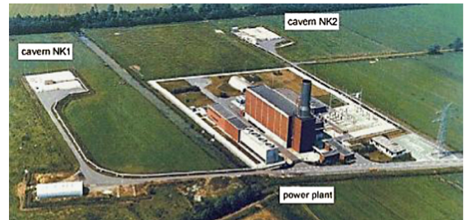
Fig. 2. CAES plant in Huntorf, Germany.
