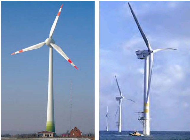
Fig. 2. Currently largest onshore wind turbine and offshore installations [8].
