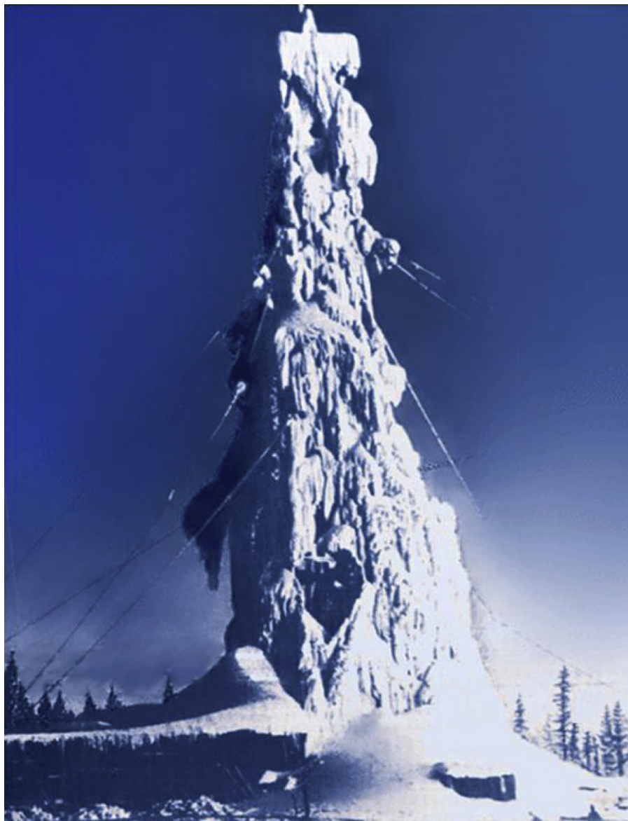
Fig. 1. The results of gas open flow at the Markha well, Yakutiya, 1963. ©Makogon.
