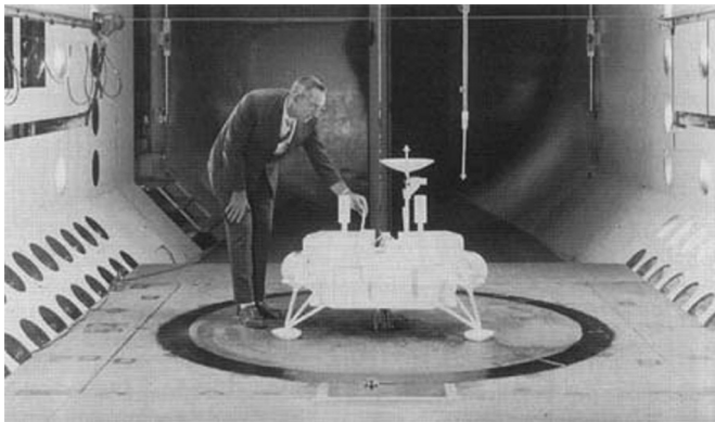
Fig. 1. A 0.45-scale model of the Viking lander is tested in a Langley wind tunnel in 1970. NASA image L-70-7351 from Hansen (1995).
