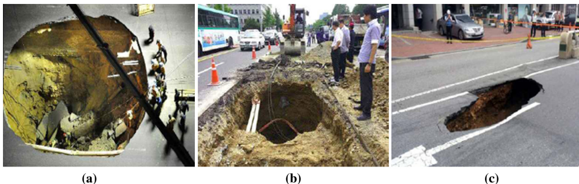
Fig. 1. Three types of human-induced sinkholes: (a) sinkhole occurred in Incheon city, Feb. 2012 by subway construction [7], (b) sinkhole occurred in front of the national assembly of Korea, June 2014 by leaking of water and sewage [8], and (c) sinkhole occurred in Songpa District of Seoul city, Aug. 2014 by construction of large building [9].
