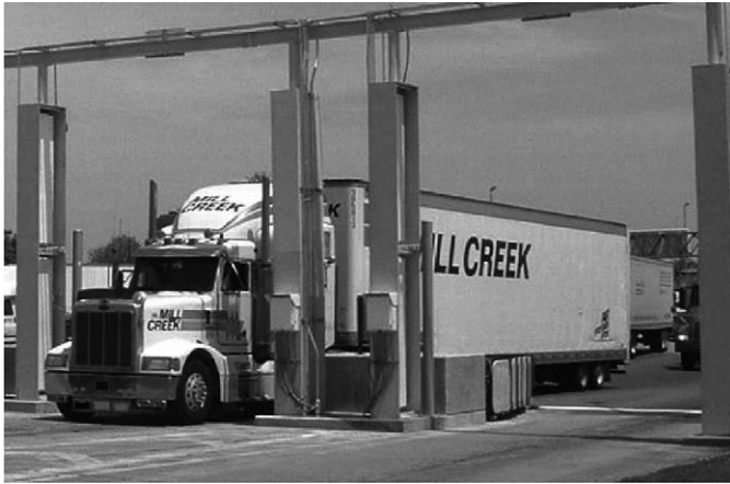
Fig. 1. A picture of a typical deployed RPM system arrangement for screening truck cargo.
