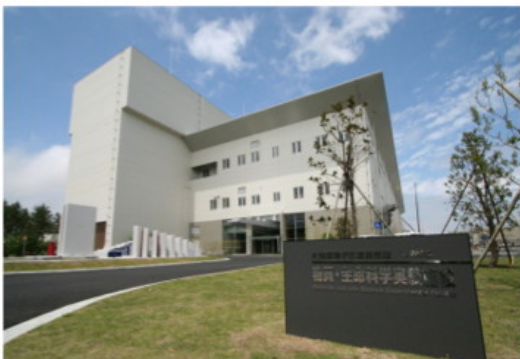
Figure 2: Material and Life science Facility (MLF).
