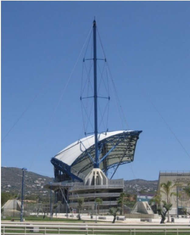
Fig. 1 – Prestressed stayed column in stadium of Algarve, Portugal [3].
