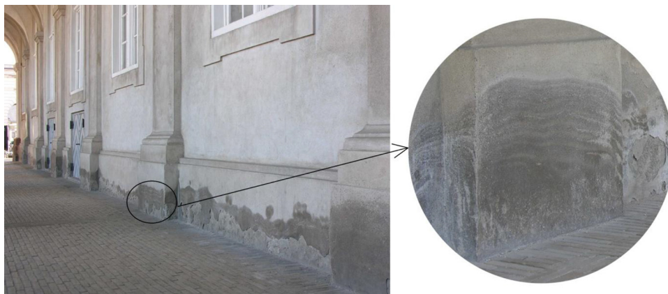
Fig. 2 – Increasing by year moisture build-up in wall.
