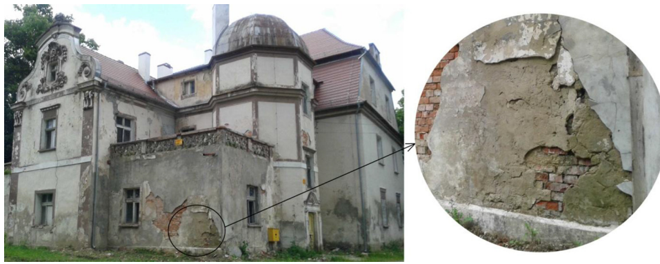
Fig. 1 – Brickwork degradation caused by excessive moisture build-up.
