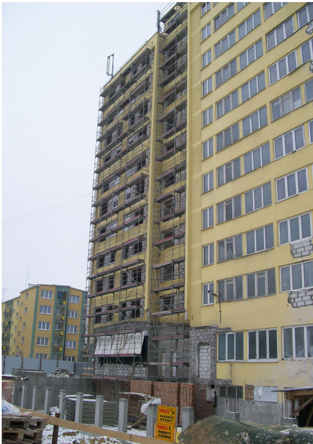
Fig. 1 – Façade scaffolding at building works in Lublin (Poland).
