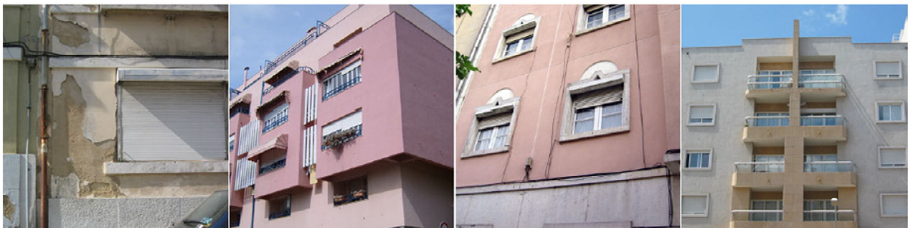
Fig. 1. Examples of the types of mortar in the rendered facades analysed: (a) lime–cement mortar; (b) current cement mortar; (c) mortar with crushed marble; and (d) single-layer mortar.
