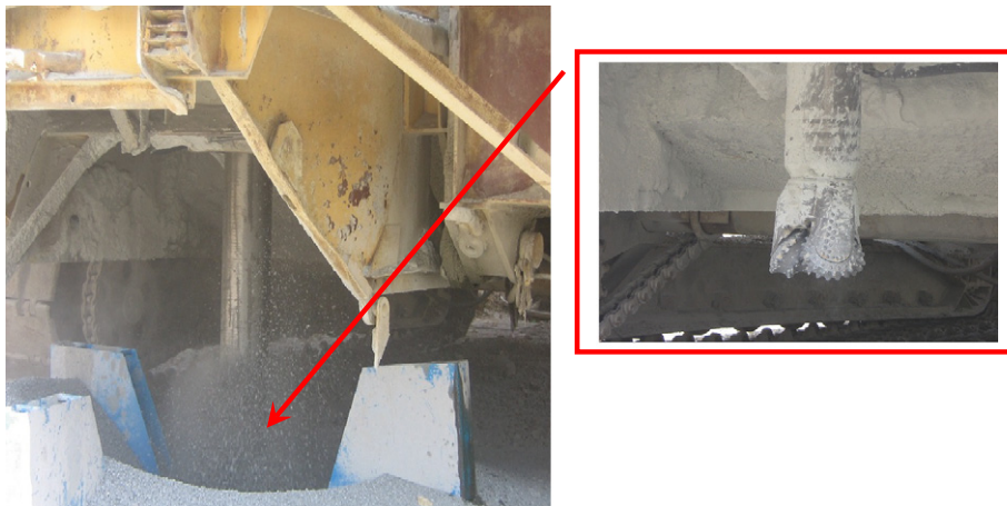
Fig. 1. Close up view of a drill bit during drilling the hole into the rockmass.
