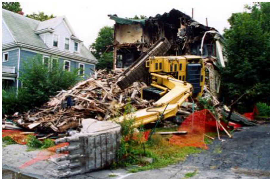
Fig. 2. Overturned excavator on building site.
