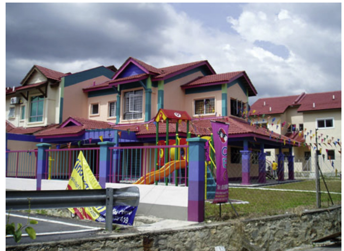
Fig. 3. Two-storey link house refurbished as a kindergarten.
