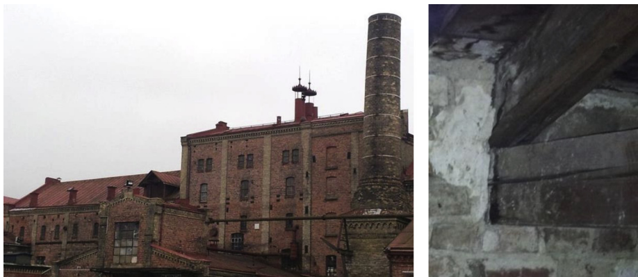
Fig. 1. Left: Lyckholms brewery in Gothenburg built in the late 1880s is listed for its characteristic exterior expression, which excludes exterior insulation as an option. Right: Connection of a wooden beam in a brick wall.
