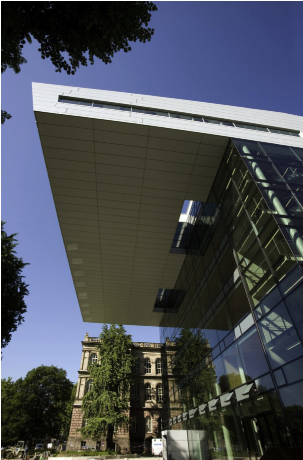
Fig. 1. Side elevation of the SuperC building. Source: RWTH Aachen university, Peter Winandy.
