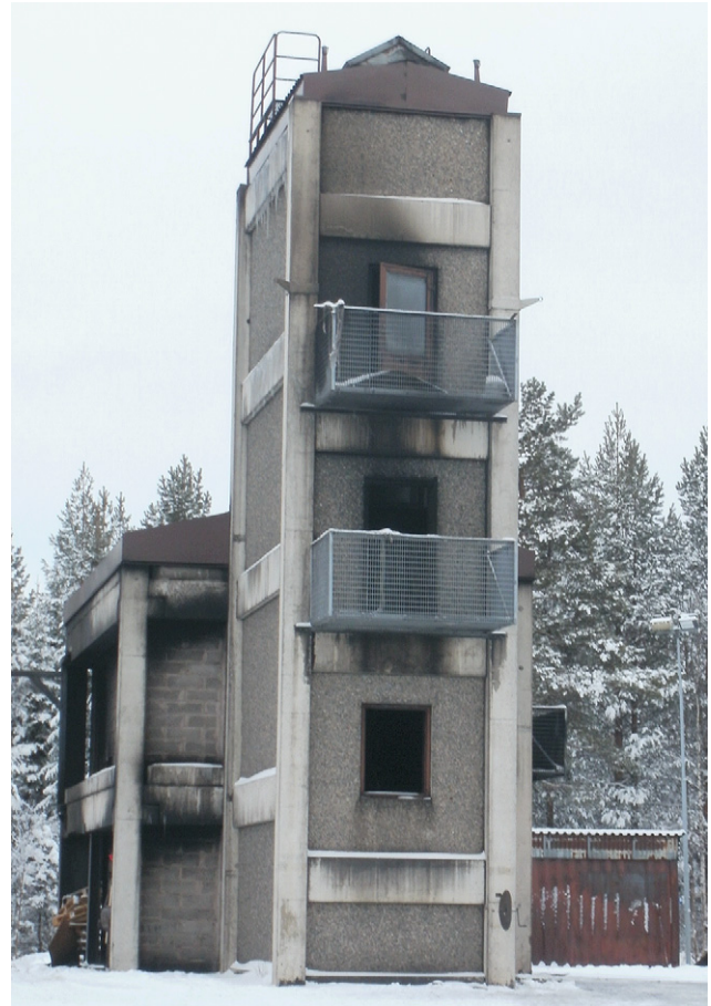
Fig. 1. Exterior of the concrete building.
