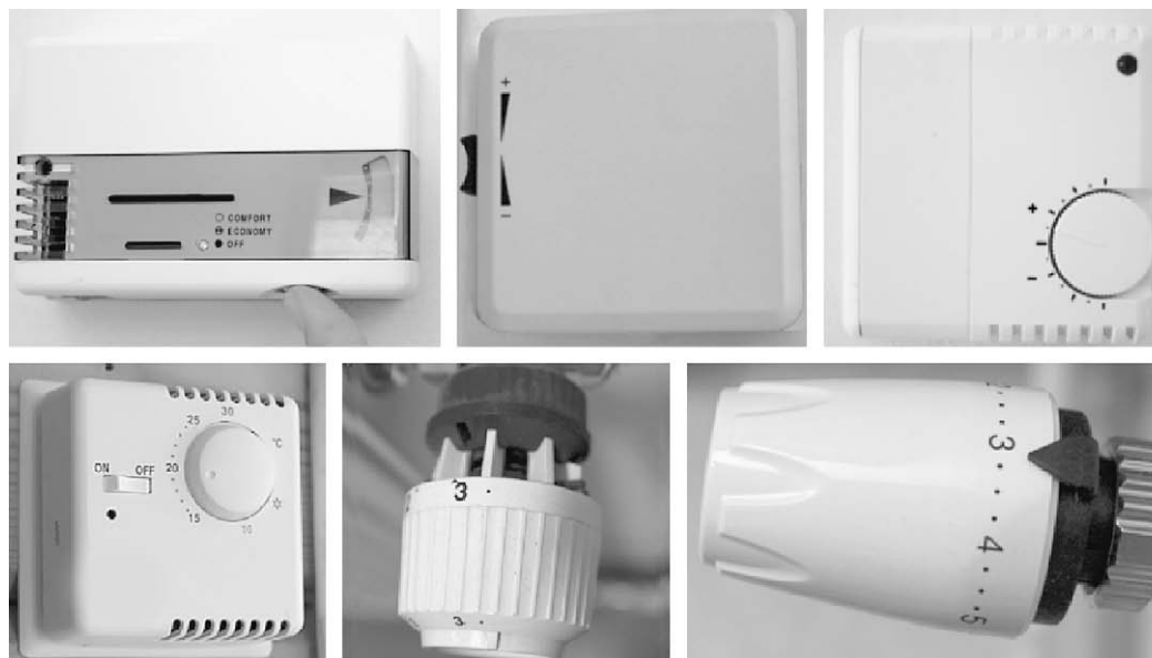
Fig. 1. Examples of typical thermostats in Finnish homes and offices. First row: room thermostats typical of offices. At left in the second row: a room thermostat typical of homes. At centre and right in the second row: thermostatic valves typical of both offices and homes.
