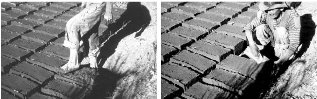
Fig. 1. Typical moulding technique of Adobe bricks ([13,14], 63).
