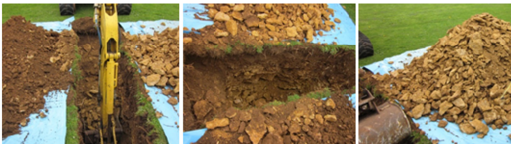
Fig. 1. Frost-shattered oolitic limestone (FSOL) unearthed during the site investigation.
