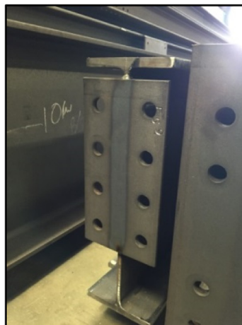
(b) Partial depth end plate
