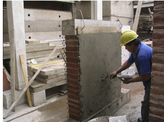
Fig. 2. Plaster application.
