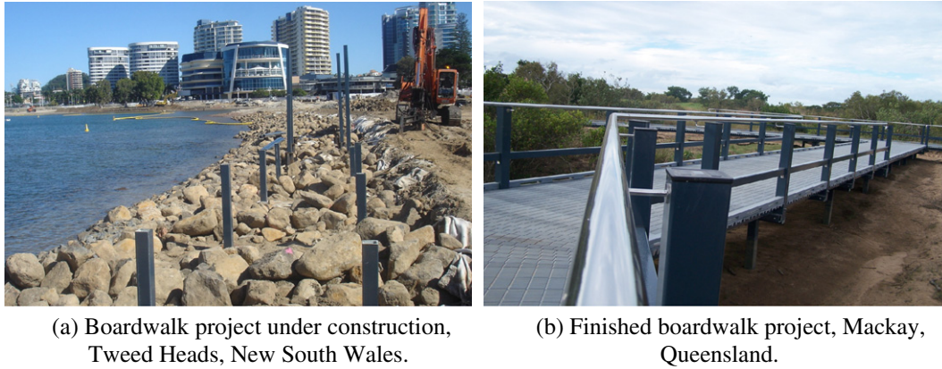
Fig. 1. Pultruded composite tubes used in shoring-up boardwalks. (Courtesy from Wagners CFT, Queensland, Australia.)
