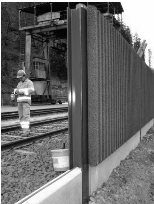
Fig. 2. GFRP post during installation of noise barrier.
