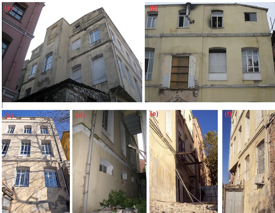
Fig. 1. Facade views of the structure the pre-restoration (a–f).
