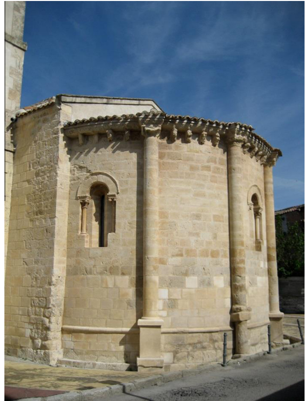
Fig. 1. Twelfth-thirteenth century Romanesque apse on church at Talamanca de Jarama, Madrid, Spain, whose upper stone ashlar is yellow and lower rough ashlar beige dolostone; occasional white limestone cladding. (For interpretation of the references to colour in this figure legend, the reader is referred to the web version of this article.)
