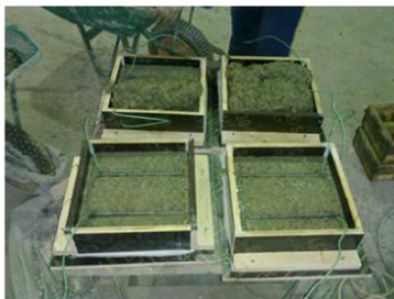
Completely filling the molds with concrete before vibration
