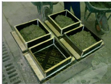
Preparation of concrete bed for steel bars
