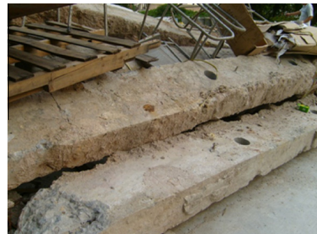
Fig. 1. Beams from waste industrial factory building.
