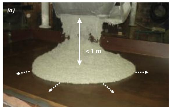
**Fig. 1.** Concrete poured from the centre of the slab and flow of concrete to the edges.
