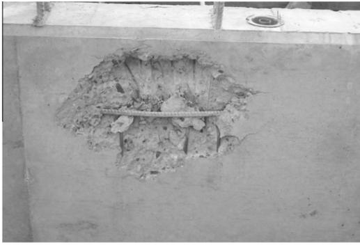
Fig. 1. Dead-end anchorage failure at the bottom soffit of slab (view from the bottom of the slab).
