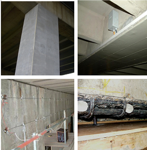
Fig. 2. Galvanic anode examples (i) a thermally applied metal coating (top left), (ii) adhesive zinc sheets (top right) [4], discrete anodes in drilled holes (bottom left) [15], discrete anodes installed in patch repair (bottom right).
